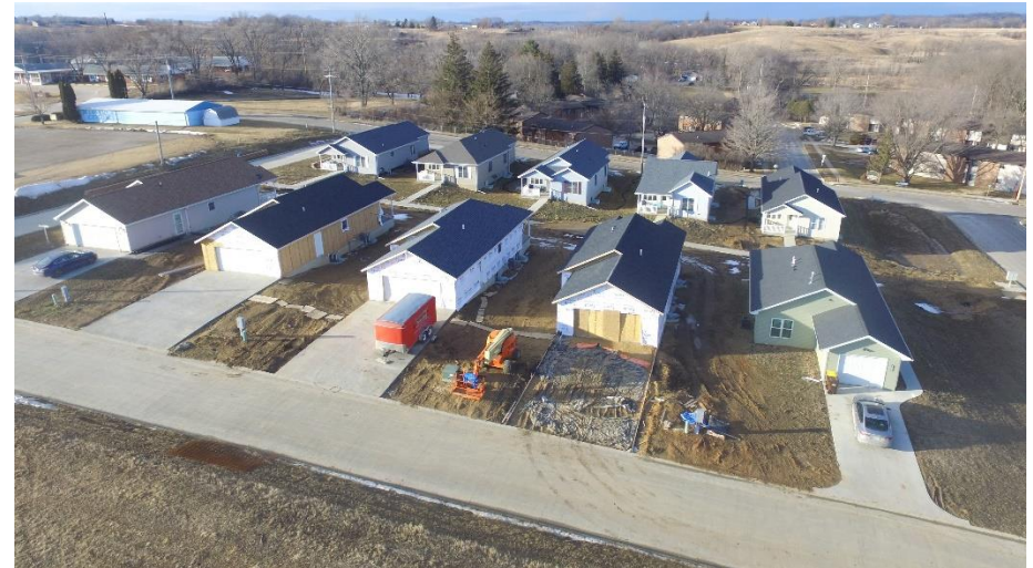
Pocket Neighborhood homes nearing completion in March 2022. The project was funded in part with Tax Increment Financing.
